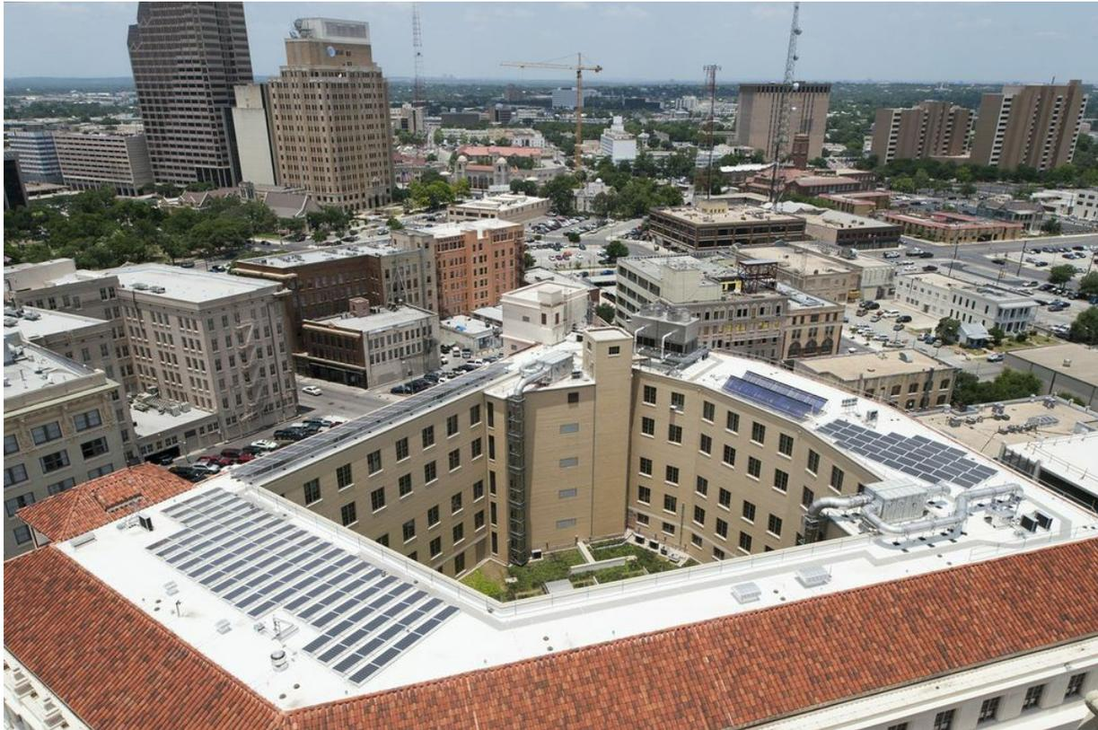
*An aerial view of the Hipolito F. Garcia Federal Building and U.S. Courthouse. Its LEED Platinum features include a green (landscaped) roof, 50 KW solar array, and energy efficient AC mechanisms. Photo by Mark Menjivar, courtesy of Ford, Powell & Carson architects.*
